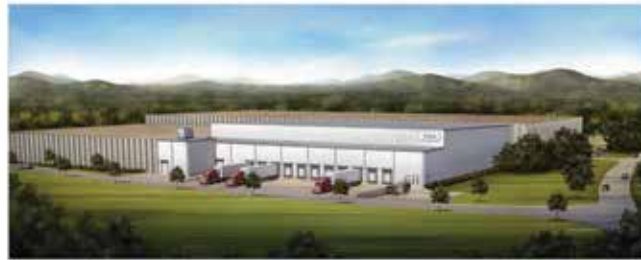
Winchester Cold Storage, Winchester, Virginia
